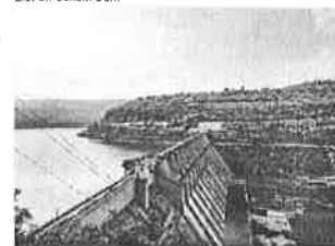
Location: Kallarhalla, Tamil Nadu, India Installed Capacity: 100 MW Operated by: TANGEDCO
